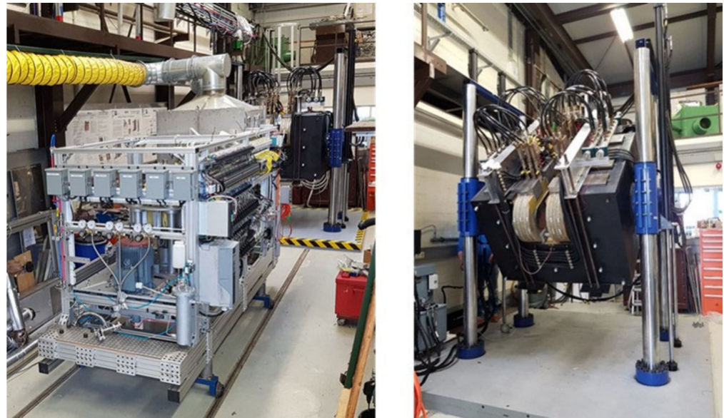
Figure 8. MaPLE PbLi loop and magnet during installation at KIT.
