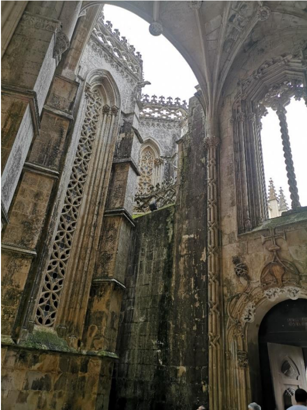
Figure 1. Bio-degradation on the inner wall of the “imperfect chapels” of the Batalha Monastery.
