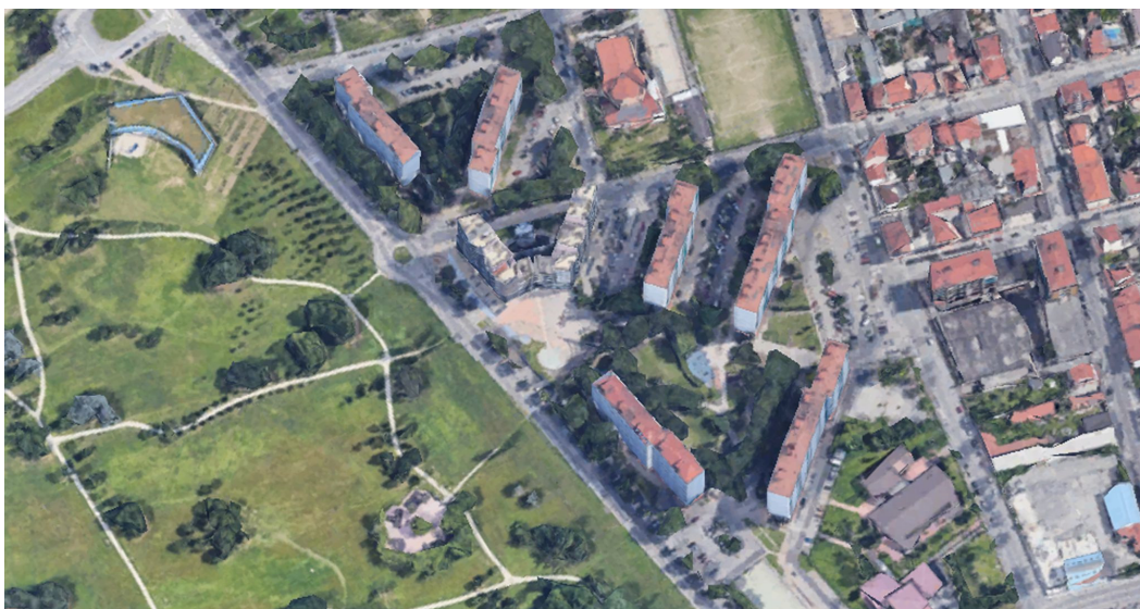
Figure 1. Via Artom public district, aerial view from Google Maps.
