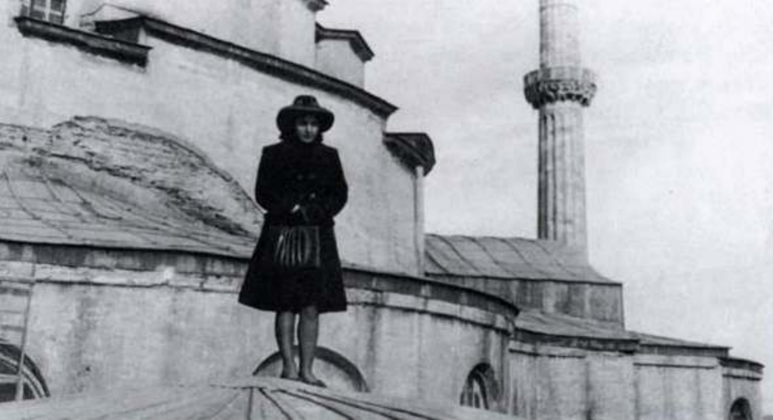
Fig. 1. Cahide Tamer, on top of one of the domes of Hagia Sophia Museum during 1956 restoration. Source: Cahide Tamer Archive, 1956, Courtesy of Virtual Architecture Museum.
