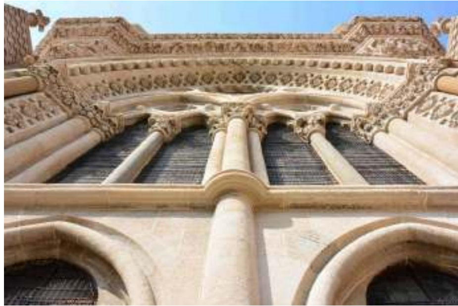
Fig. 2. Rajabai Clock Tower. Courtesy of SNK Architects.
