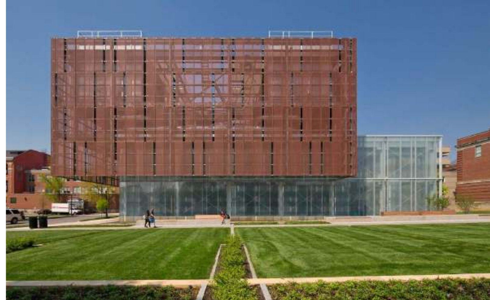
Fig. 1. Leers Weinzapfel Associates, The Ohio State East Regional Chilled Water Plant Columbus, Ohio, USA, 2015. © Photograph Leers Weinzapfel Associates.
