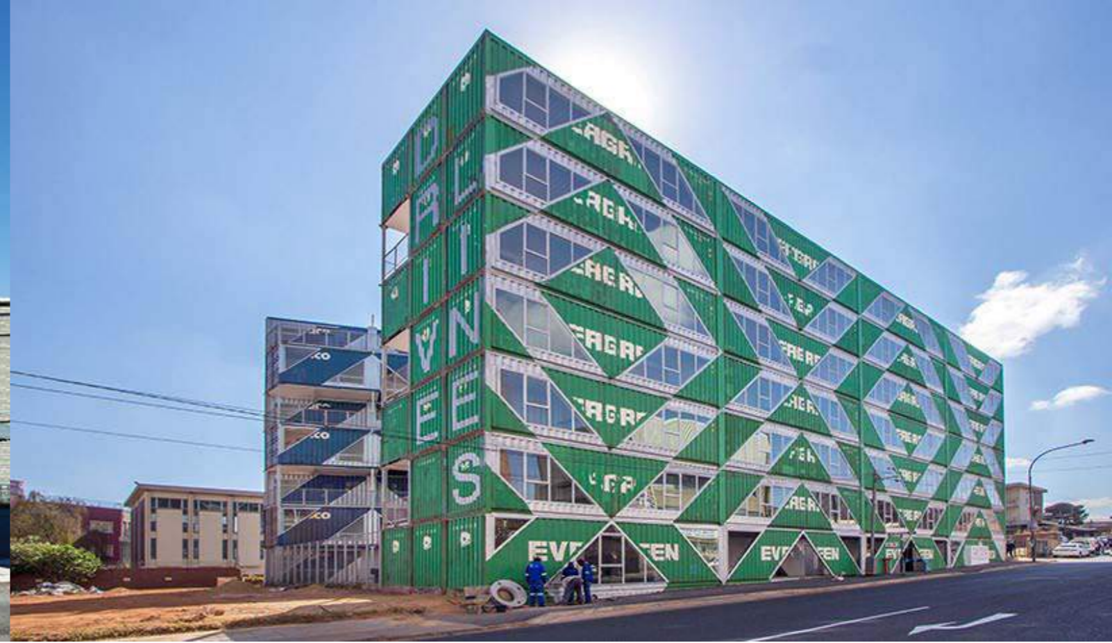
Fig. 2. LOT-EK's Drivelines residential-studios and retail building resembling the ancient Mayan technique of binding discarded recyclable materials, Johannesburg, South Africa, 2014-17. Photo: Danny Bright. Source: http://www.lot-ek.com/filter/residential/DRIVELINES-STUDIOS .
