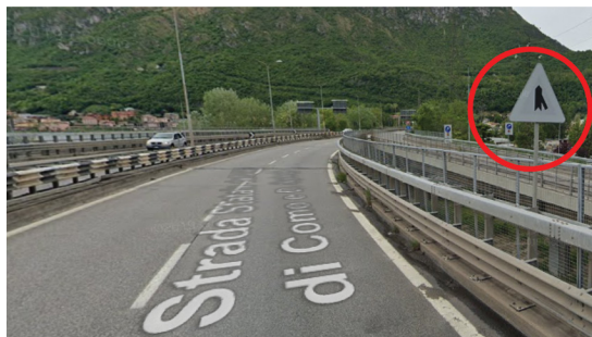
Figure 7: Example of not fully visible vertical road sign, close to the merging ramp. Source: www.google.it/map.
