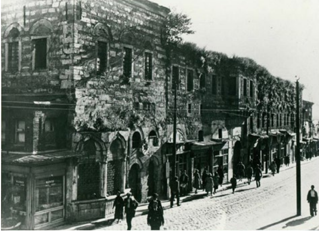
Figure 5. Istanbul. Simkeşhane, 20 th century. Ataturk Library, Husrev Tayla Archive, Accession N. FOTO_019084. The fountain can be seen on the corner of the building facing the street on the far left. The types of shops on the ground floor, the poor condition of the units on the first floor and the heavy vegetation on the roof suggest that the building was already in a poor condition in this period and the simkeş craftsmanship had already waned. The shop on the bottom left of the photograph reads “ manav ”, which means greengrocer. The clothes of pedestrians (men in suits with hats, women without headscarves and with skirts) and the use of Latin script for “ manav ” indicate the photo was taken after 1928. A tram line is also visible on the street. This was constructed in 1914 in the second constitutional era of the Ottoman Empire (1914-1918).
