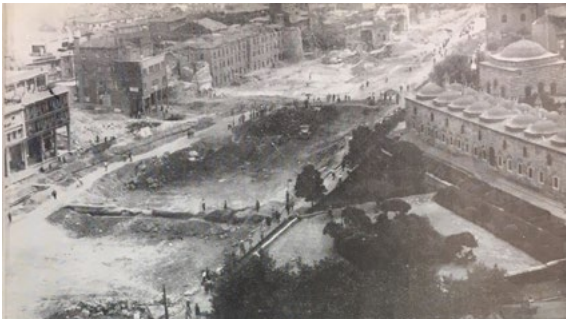
Figure 19. Istanbul. Ordu Avenue during the demolition (from Istanbul'un Kitabı 1957, p. 35).
