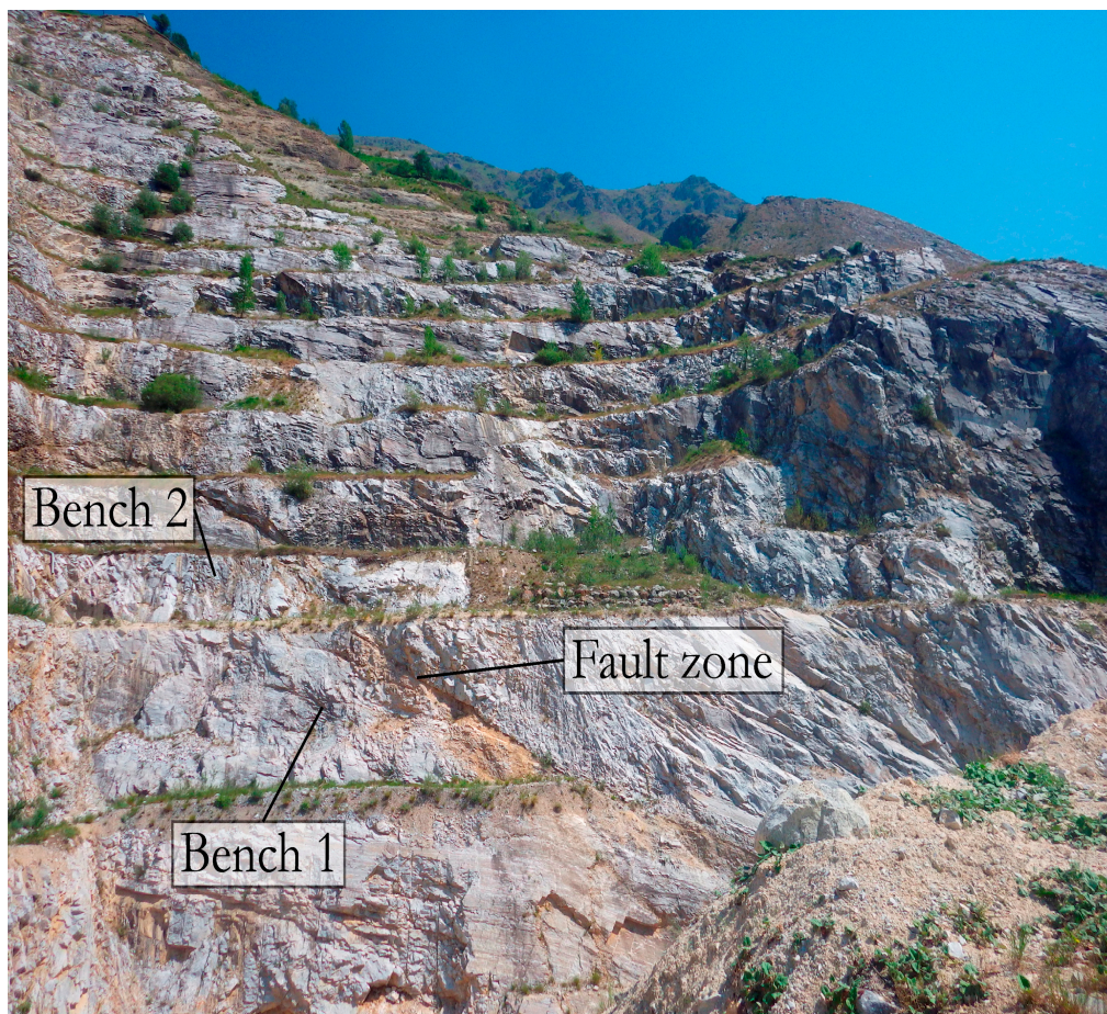
Figure 1. Overall perspective of the test site.
