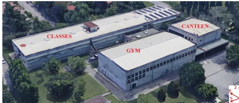
Figure 1. Aerial view of the specimen structures
