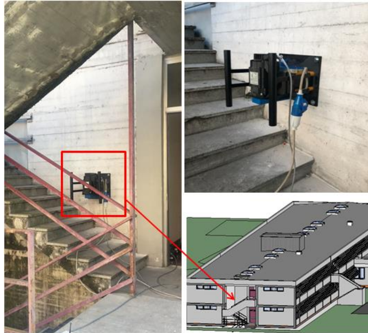
Figure 5. Vibrodyne position on the shear wall
