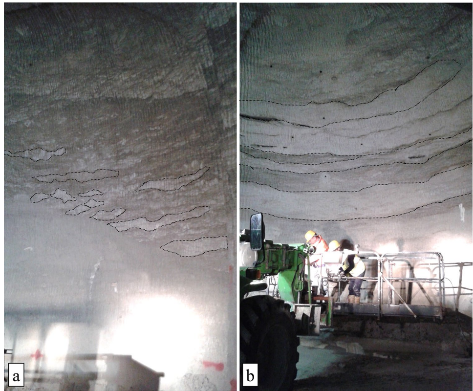
Fig. 27 Excavation faces in underground tunnels in branching selenite gypsum with different macro-textural features. a Small gypsum nodules in a predominant fine matrix. b Big coarse gypsum branches with lower concentration of finer matrix
