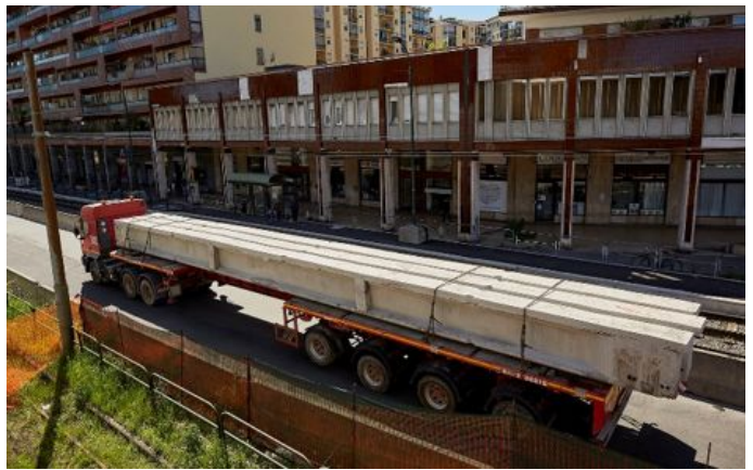
Figure 11. PC beams transportation phase.
