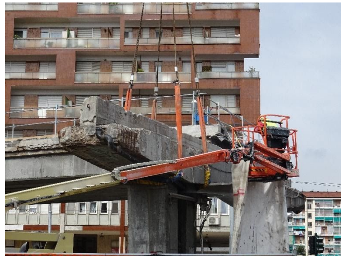
Figure 10. Dismantling phase of pier caps.
