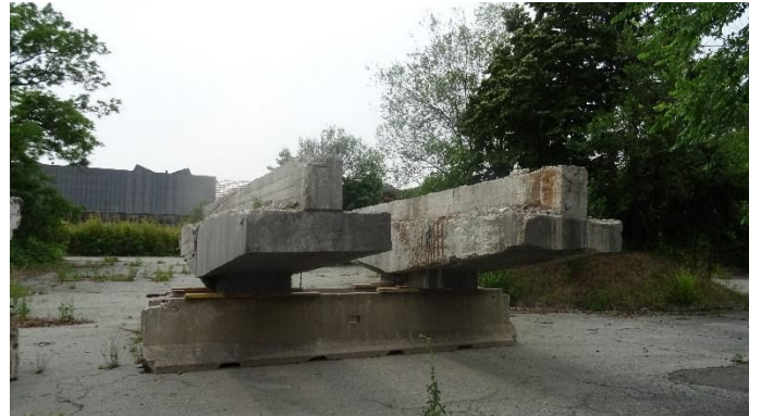
Figure 15. Pier caps located in the testing site.
