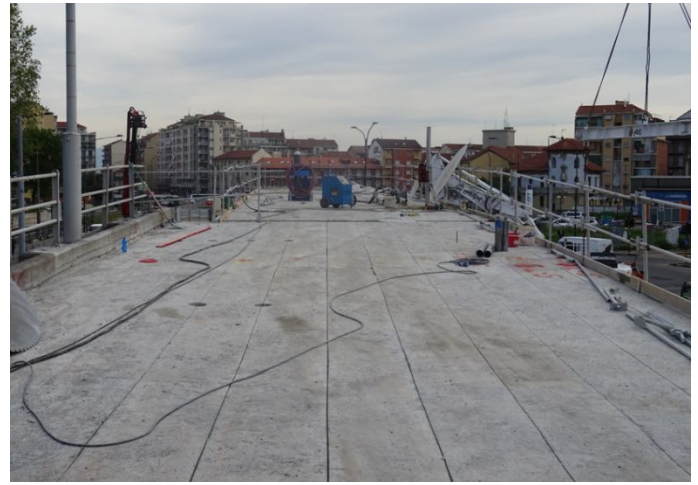
Figure 7. Concrete beam cutting phase.
