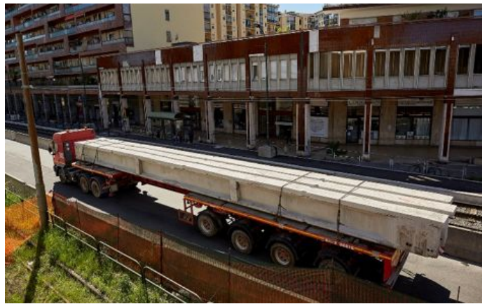
Figure 11. PC beams transportation phase.
