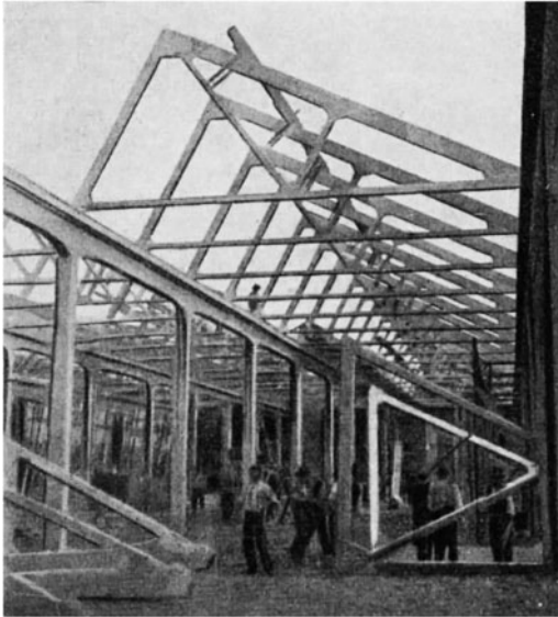
Figure 2. Assembly operation of the reinforced concrete truss girders, previously prefabricated on the ground (Santarella 1931: 346).
