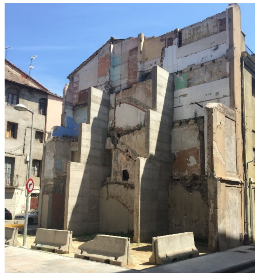
Figure 8. Unparelldarquitectes, Situation after the demolition, 2017 © unparelldarquitectes.
