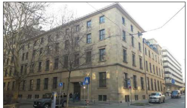
Fig. 2: Building 2 of HFT Stuttgart
