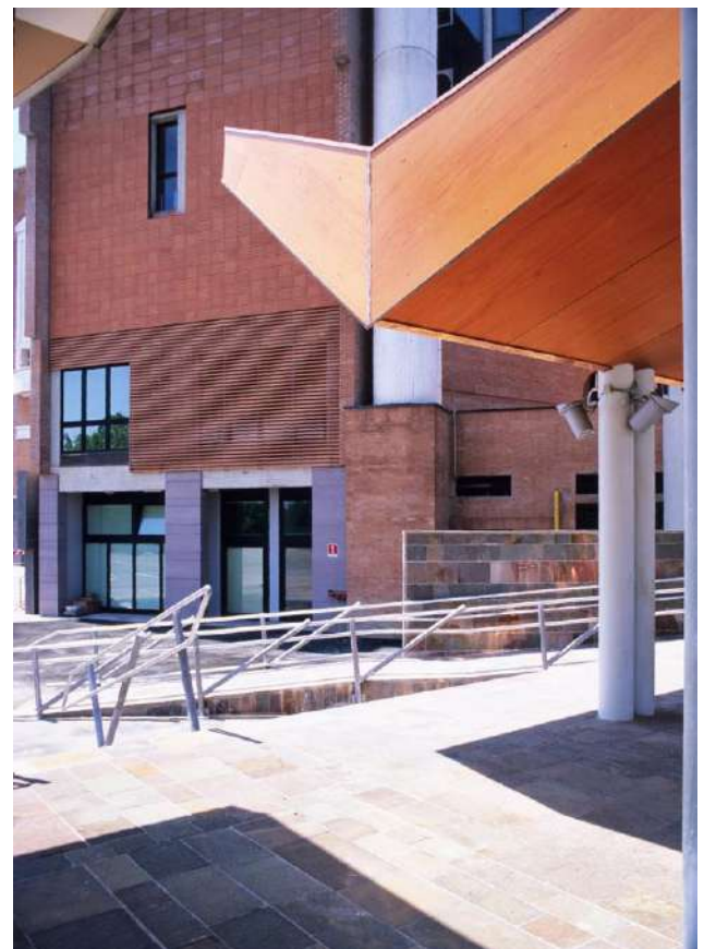
Fig. 13: New railway station of Zola Predosa (BO)
