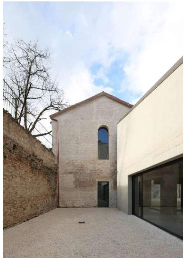
Fig. 13: the courtyard behind Laboratories - Ph. Schulte Bunert
