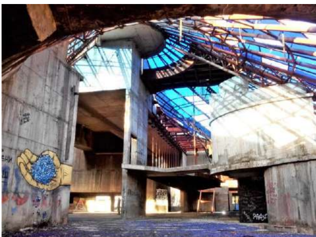
Fig. 17: Interior spaces, today
