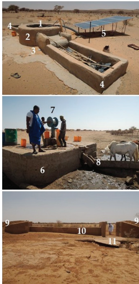
Figure 12. Open well (1) showing low apron (2) and basement (3), water trough for cattle watering (4), solar panels (5) in Boukhzama 1; a well provided with raised basement (6), a manual water pump (7), and a broken water trough (8); an earth embankment (9) provided with spillway (10) and lock (11) in Agoueinit.
