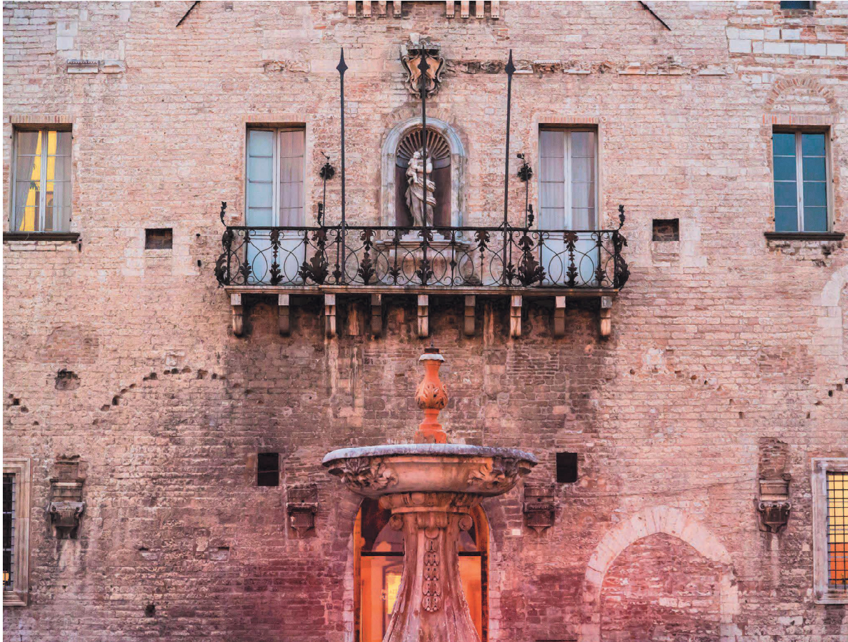
Figure 1 | Cagliari, town hall. Source: © Andrea Tessadori
