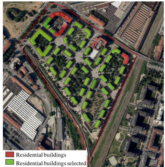
Figure 5. Arquata district with residential buildings
