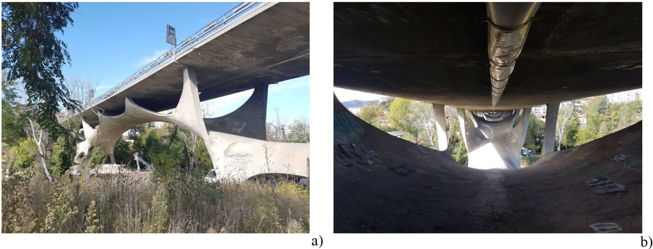
Figure 1: Basento Bridge in Potenza, Italy (Photos: Carlo Atzeni)
