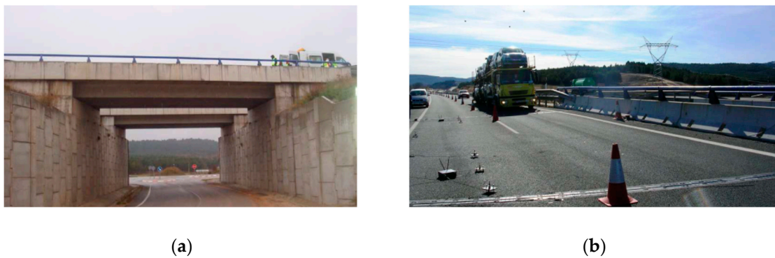
Figure 1. The skewed highway bridge: (a) Side view; (b) front view (during the measurements).
