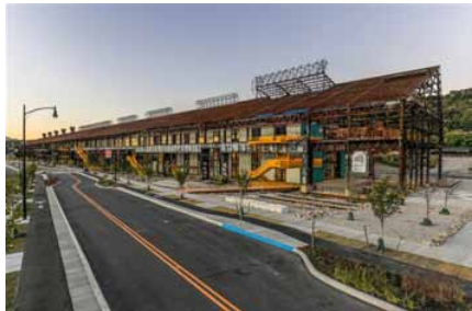
Figure 4. Hazelwood Green, Mill 19, Pittsburgh. Source: (Turner construction services. 2019)
