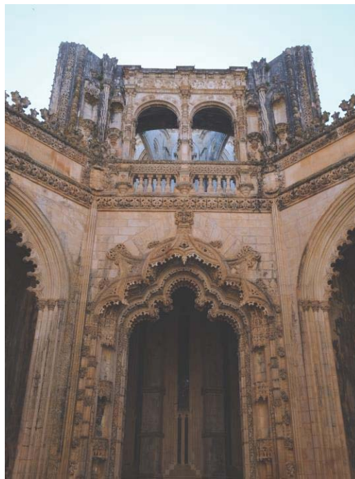
Fig. 1. Facade and sculptures with orange patina at the Imperfect Chapels, Batalha Monastery.
