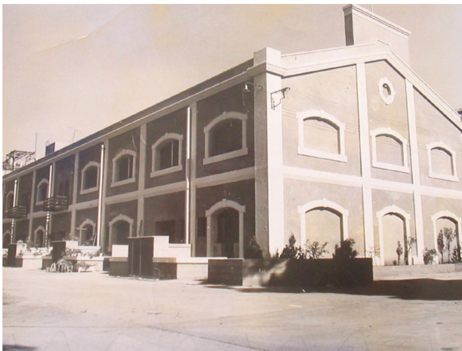
Fig. 6. Apartments integrated into the original factory (photo at the end of the works). All the openings have been respected; only wooden balconies have been added; in front of each entrance a small private garden enhances the sense of privacy.
