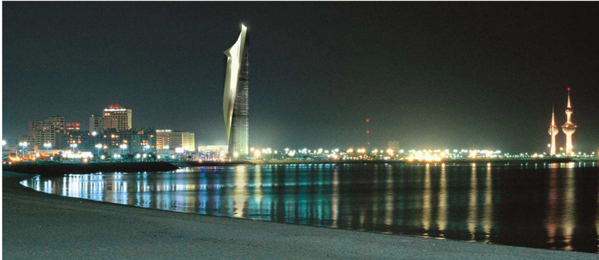
Figure 6: Image of the Al Hamra tower.
