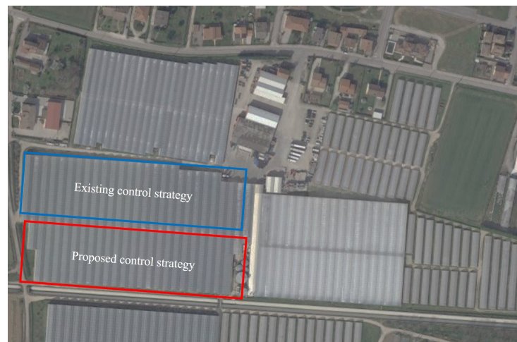
Figure 1. Overview of the greenhouse where the experimental setup was installed.
