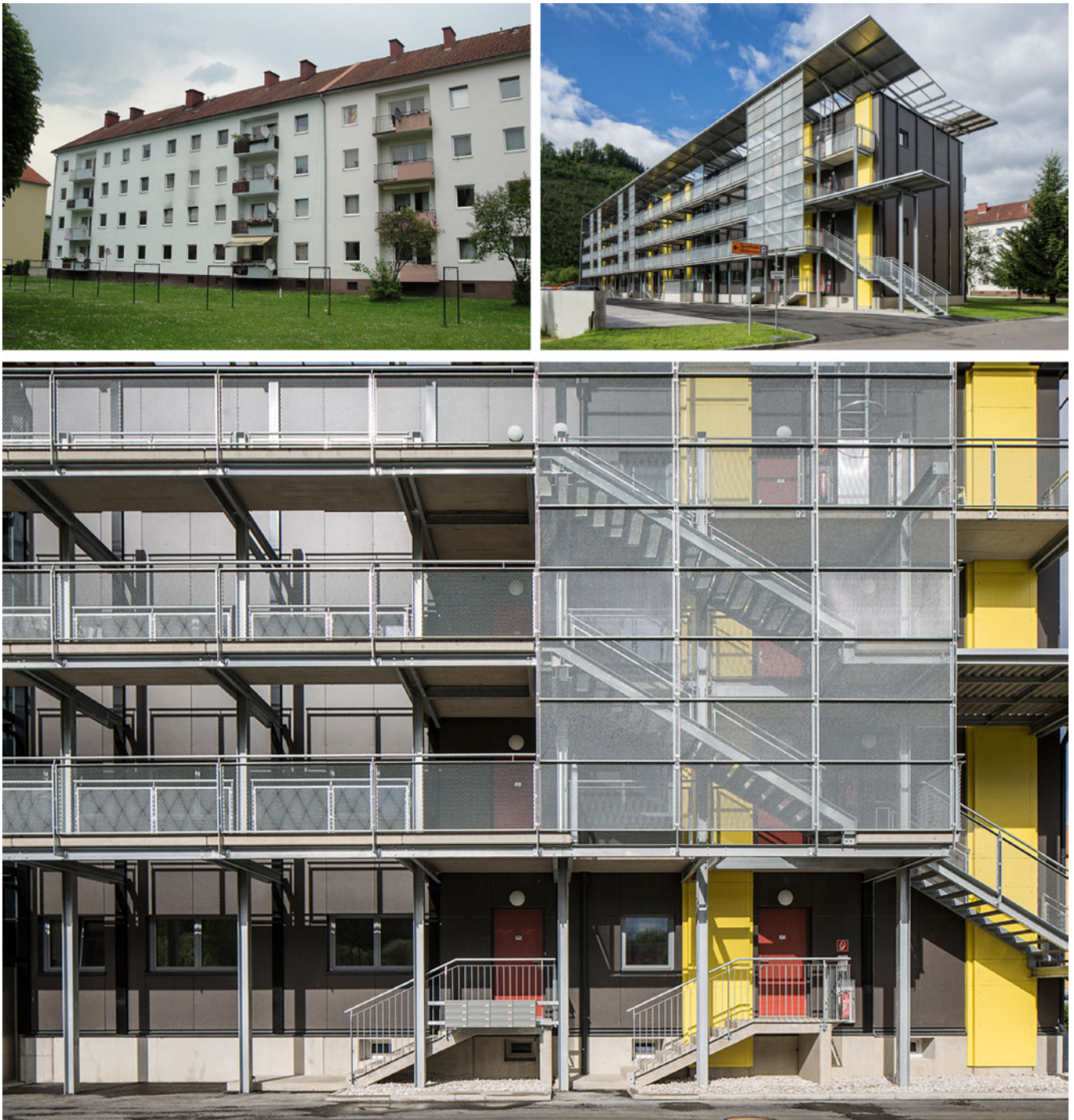
Fig. 3. Post-war residential building (built in 1960-1961) in Kapfenberg (Austria) before (a) and after renovation (b); Rear counter-façade with new spatial arrangements (c). Source: https://architizer.com/projects/renovation-residential-building-kapfenberg/ .
