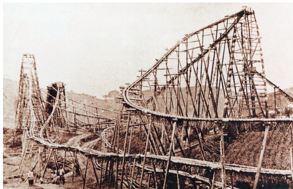
Figure 7.1: Replication of the transport system through bamboo pipelines used to transport natural gas [77].
