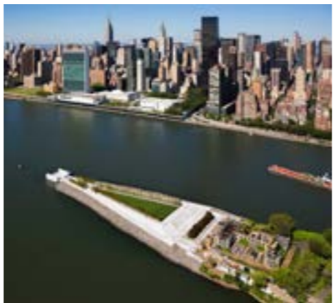
Aerial view with Manhattan in the background (above). ( https://www.mitchellgiurgola.com/portfolio/projects/franklin-d-roosevelt-four-freedoms-park/ )
