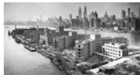
View of the Goldwater Memorial Hospital under construction (1939, www.underwoodarchives.com).
