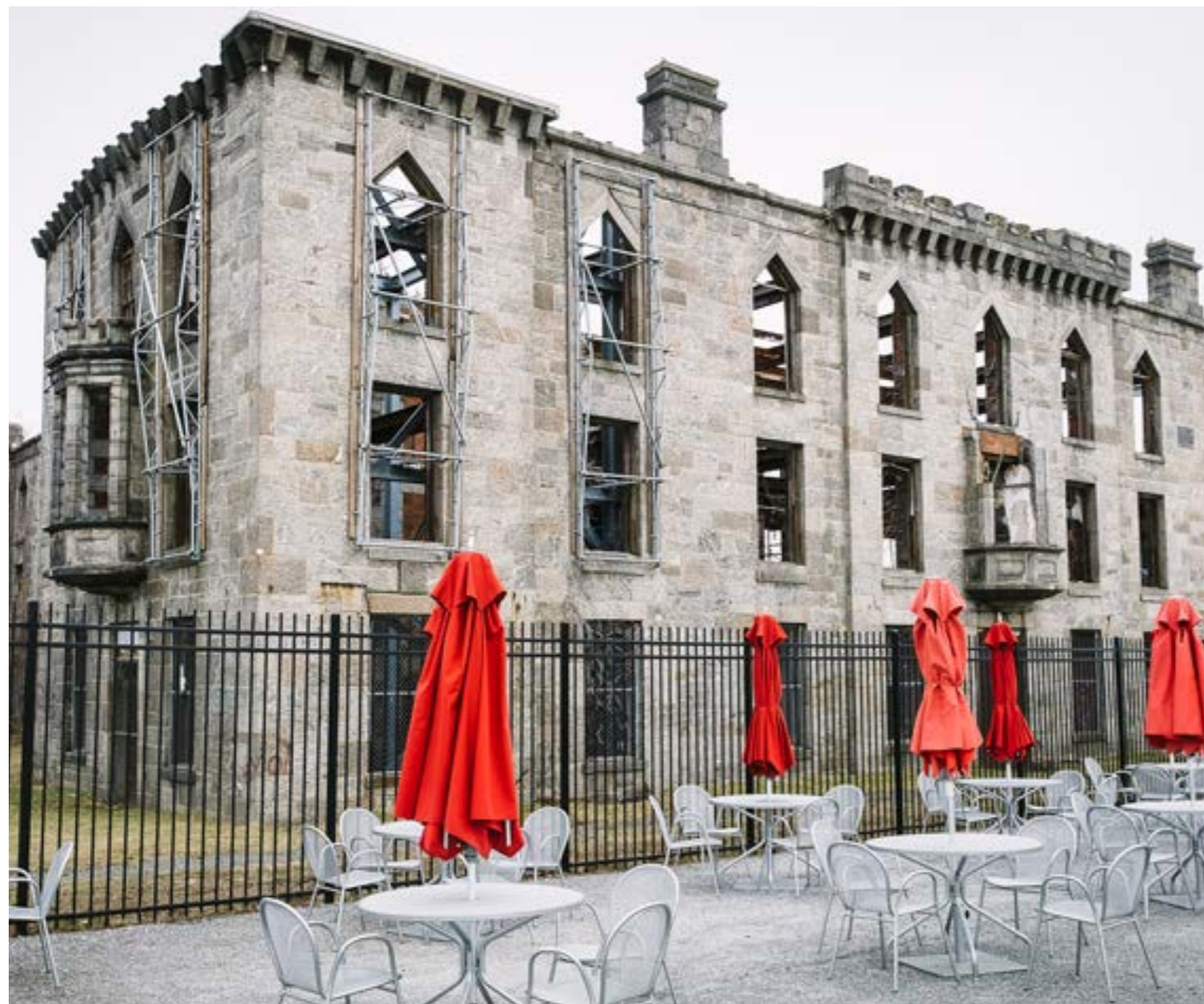
Smallpox Hospital, southern façade (2017, Balocco, Iurlaro, Lauri, Ravizza).
