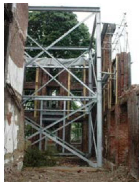
Interior of the northern wing after stabilization (2009, John Milner Associates).
