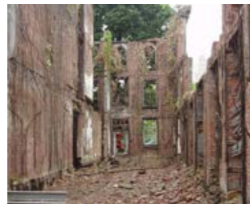
Interior of the northern wing before stabilization (2009, John Milner Associates).
