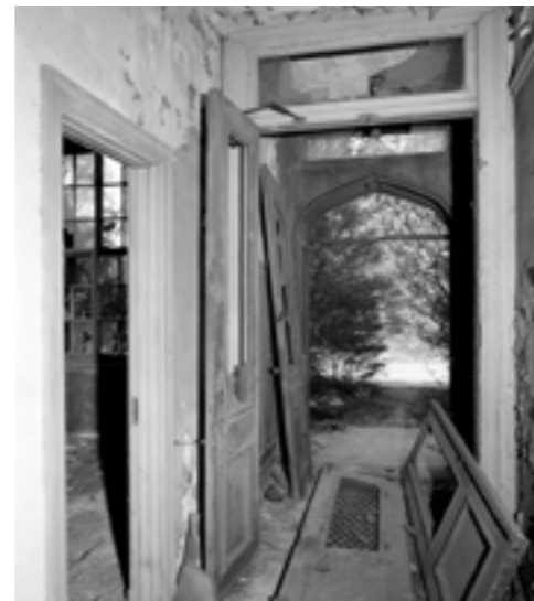
Interior hallway and entrance, the interiors of the building no longer exist, 1983 ( https://www.theruin.org/history ).
