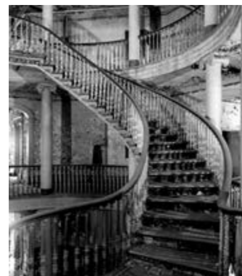
The Octagon, view of the helical staircase, in a state of neglect, 1970 ( https://www.theruin.org/blog/2016 ).
