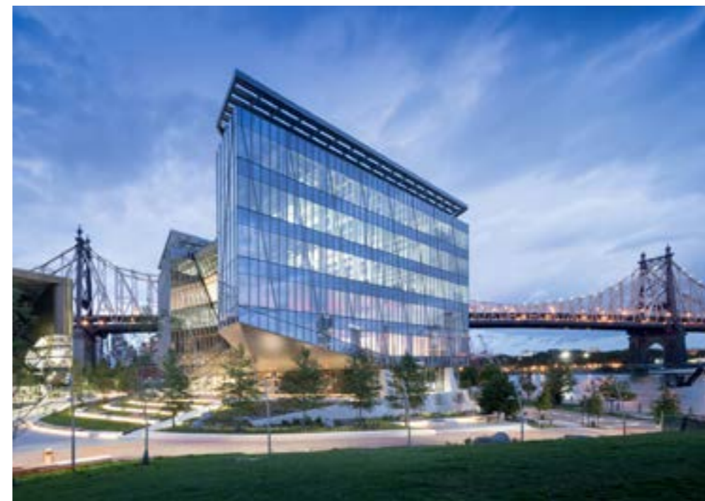
View of a Tata Innovation Center cantilevering part, also known as The Bridge. ( https://www.theplan.it/eng/award-2019-education/tata-innovation-center-at-cornell-tech )
