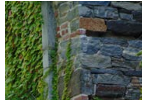
Eastern façade, detail of the internal wall (2017, Balocco, Iurlaro, Lauri, Ravizza).
