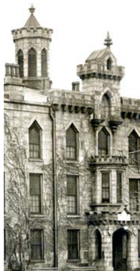
Smallpox Hospital, detail of the western façade (after 1905, www.theruin.org).
