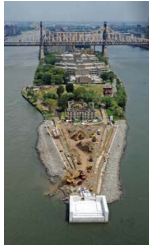
The FDR Memorial under construction. ( https://sciame.com/portfolio/franklin-d-roosevelt-four-freedoms-park/ )
