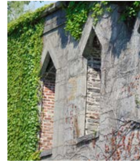
Masonry detail of the eastern façade (2017, Balocco, Iurlaro, Lauri, Ravizza).
