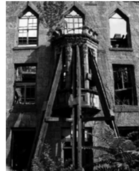
Consolidation works, western façade, project G. Cavaglieri (after 1970, www.theruin.org).
