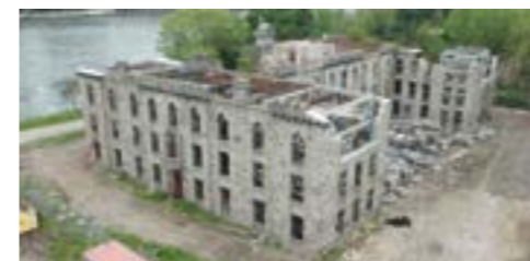
Southern view - east of Smallpox Hospital ruin after stabilization (2009, John Milner Associates).
