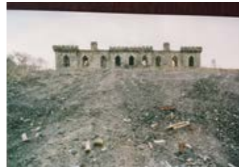
Southern façade partially obscured by the accumulation of excavated material (1960-69, Archive Roosevelt Island Historical Society).
