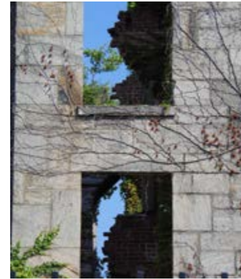
Western façade, external cladding slabs (2017, Balocco, Iurlaro, Lauri, Ravizza).
