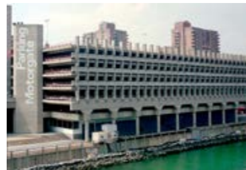
View of the Motorgate Garage from the East River. ( https://www.nycurbanism.com/brutalnyc/2017/2/15/eastwood )
