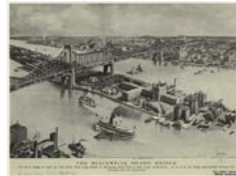
The Blackwells Island Bridge (1861-1903, New York public Library, online Archive).
