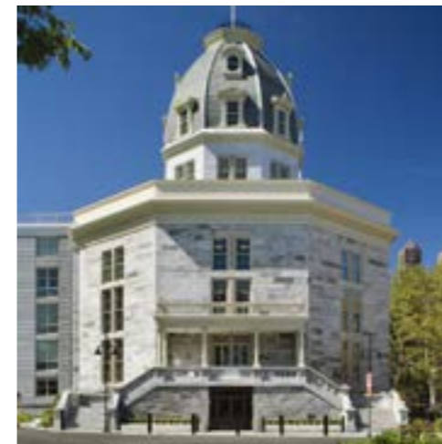
The Octagon after the renovation as the main access to the new residential complex ( https://www.beckerandbecker.com/work/octagon ).
