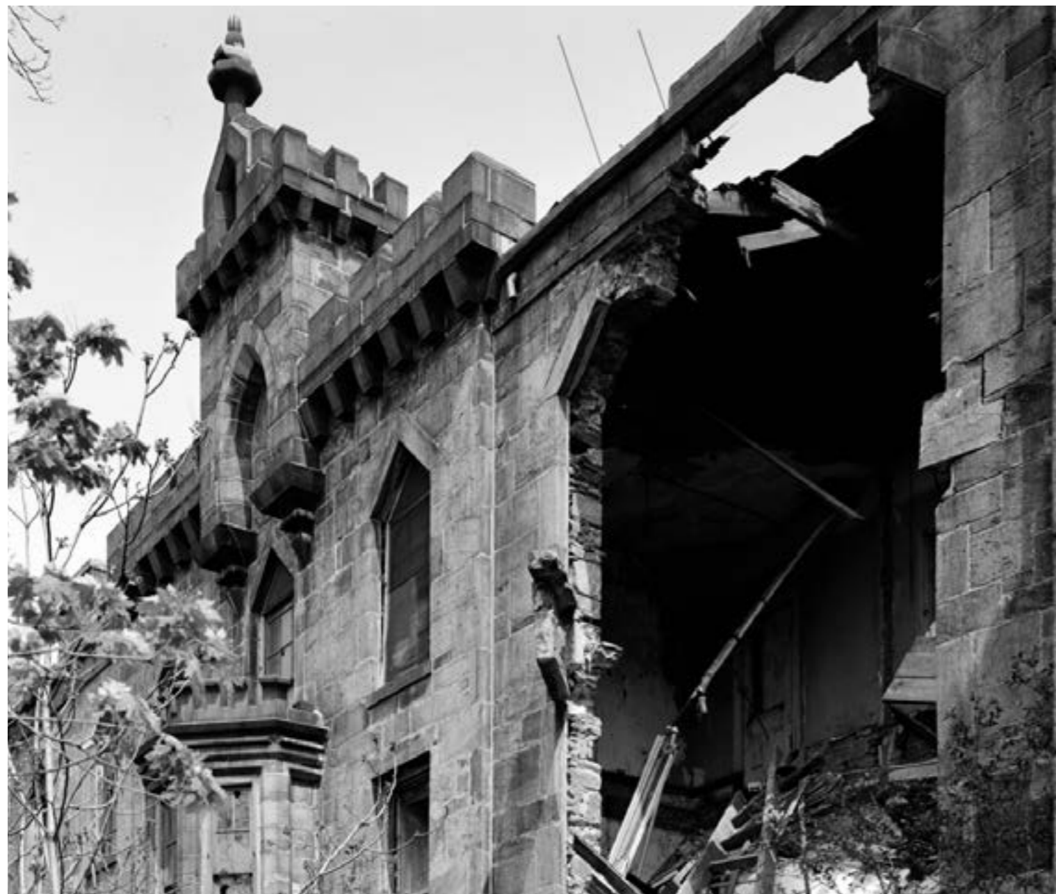
Western façade showing a partial collapse of the wall, Library of Congress, 1983. ( https://theruin.org/history ).
