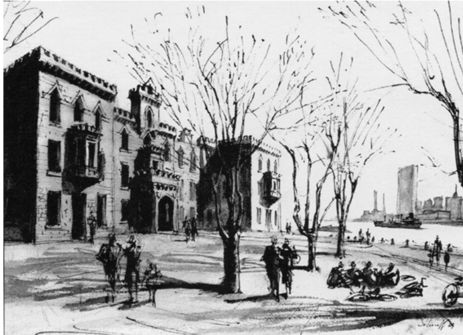
Smallpox Hospital, sketch of the western façade (1969, J. Berdy, Roosevelt Island. Images of America, Charleston, SC, 2003, p. 121).
