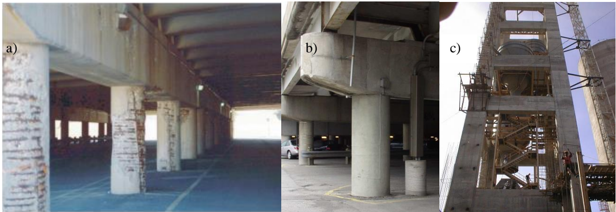
Figure 12 Highway bridge damaged by steel corrosion (a), Rehabilitated columns after twenty years of service (b), deficient industrial structure (c)
