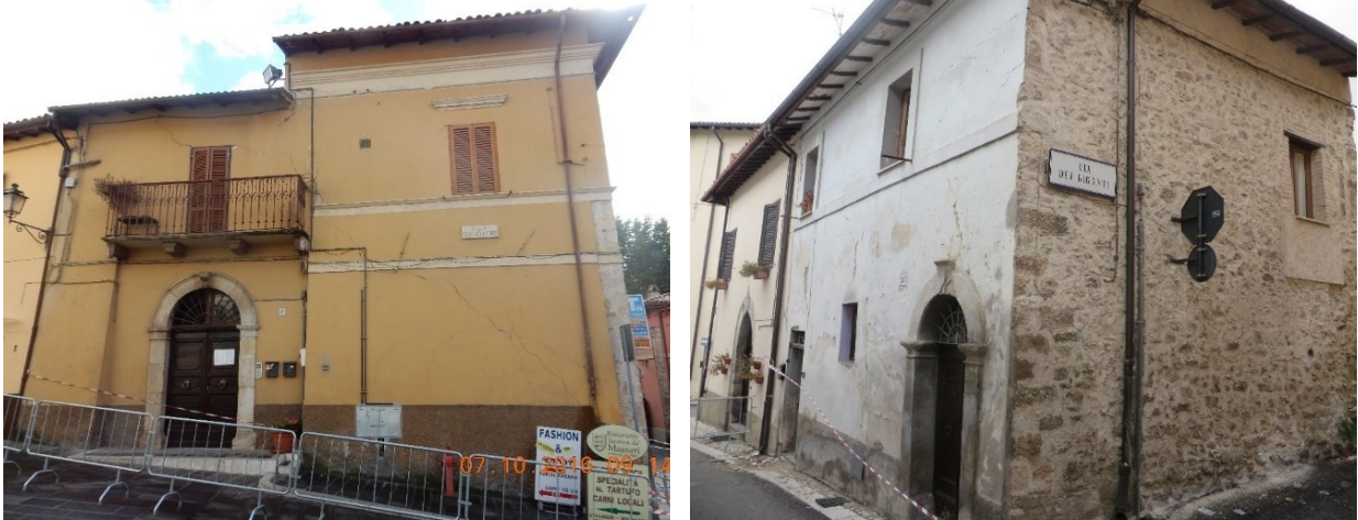
Figure 5.33. Limited damage was observed in the buildings of Norcia.
