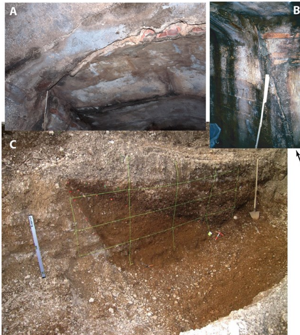
Figure 2.5. Norcia fault: emergence of active fault splays in the settled area of Norcia: a, b) vault and walls of a cellar displaced by a fault which activated during the earthquake of 1979; c) panoramic view of the trenches excavated by Galli et al. (2005) in the suburbs of Norcia: the fault places Middle Pleistocene alluvial gravels in contact with colluvial units ranging in age from the Upper Pleistocene (i.e. the lowermost unit with the orange matrix in the hanging wall) to the 18th century AD.
