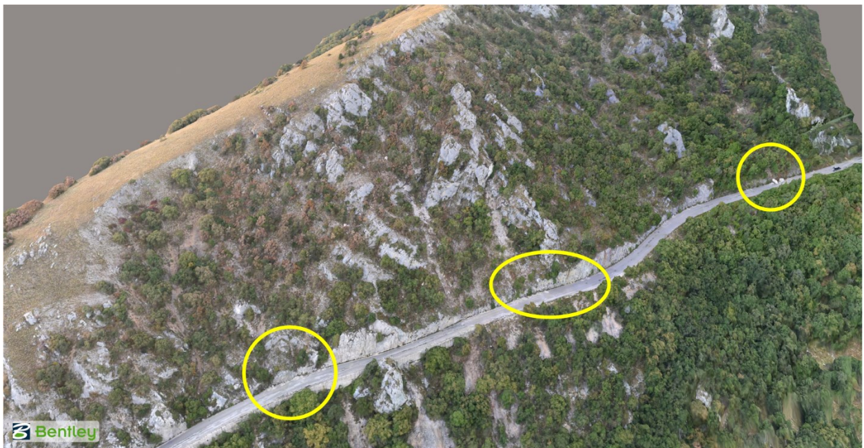
Figure 4.19. 3D model image of the SP 477 rockfall. Visible rocks and debris on the road are circled in yellow (42.7661 N 13.1669 E).
