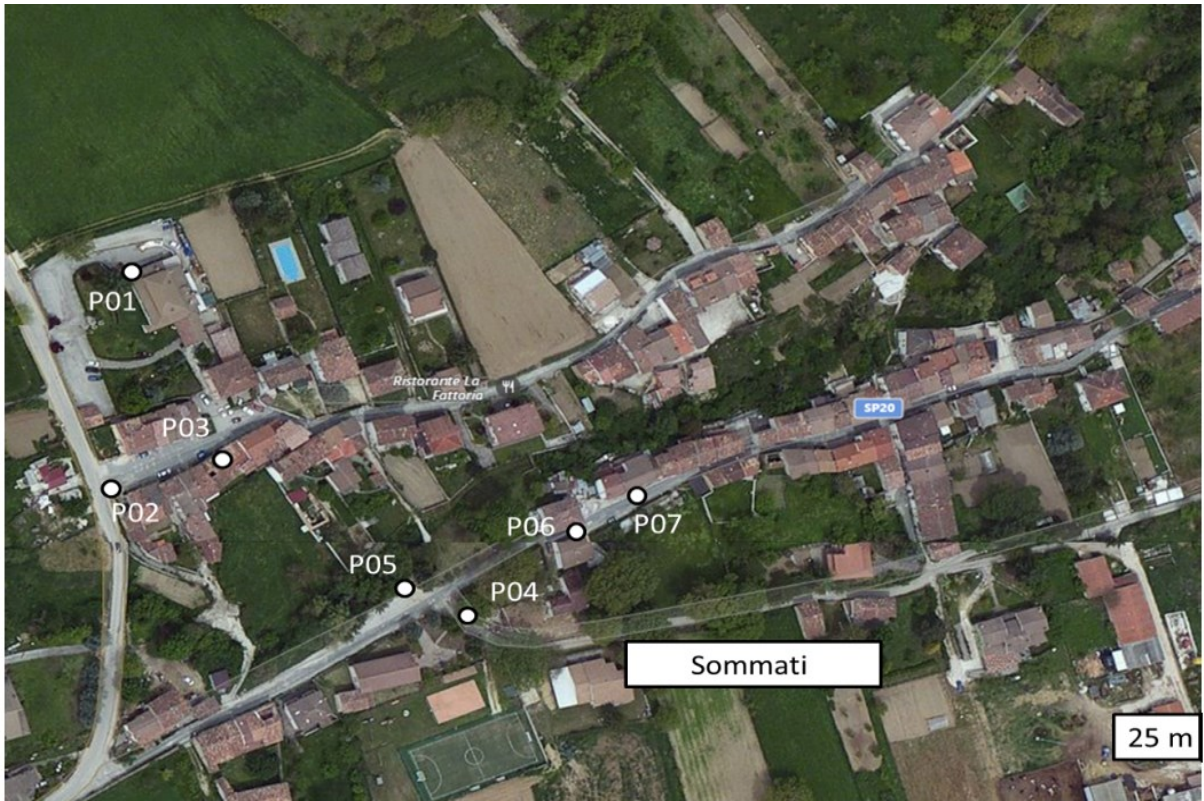
Figure 5.69. Locations of representative structures inspected in Sommati (see Table 5.18 for details).
