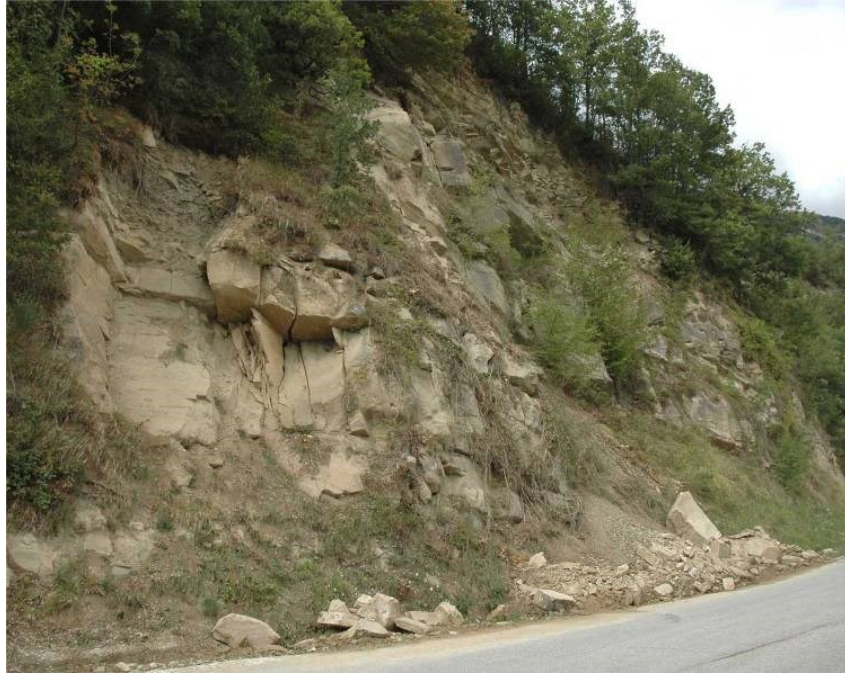
Figure 4.6. Free-face wedge sliding that is governed by bedding joint attitude.
