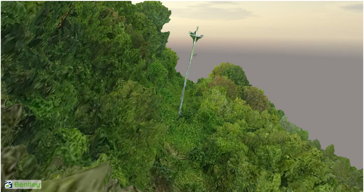
Figure 4.46. 3D model image of a rotated telephone pole in the slope below the cracks. The telephone pole is rotated 13 degrees from vertical, while the other telephone poles are approximately vertical.
