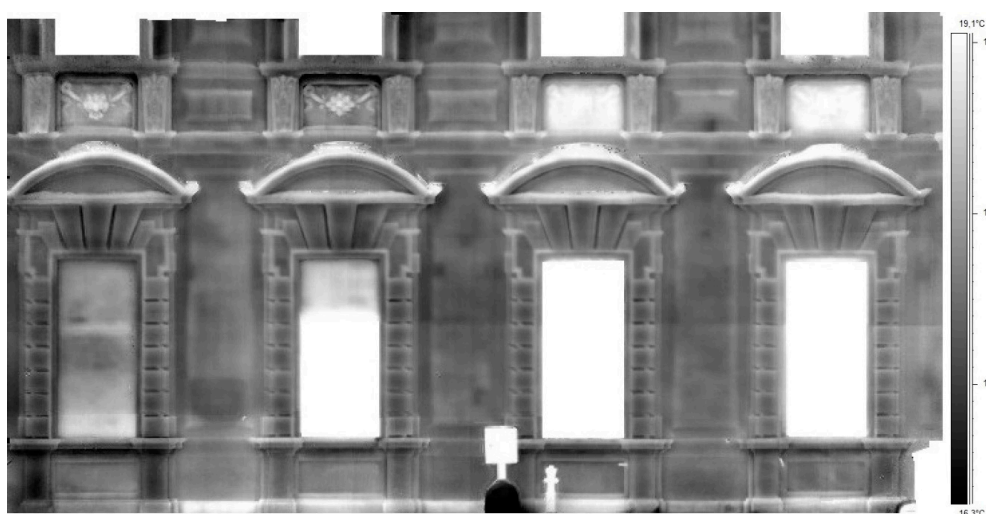
Figure 13. Thermal orthophoto-mosaic produced with FLIR 660SC imagery.
