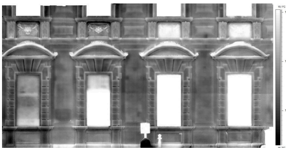
Figure 13. Thermal orthophoto-mosaic produced with FLIR 660SC imagery.
