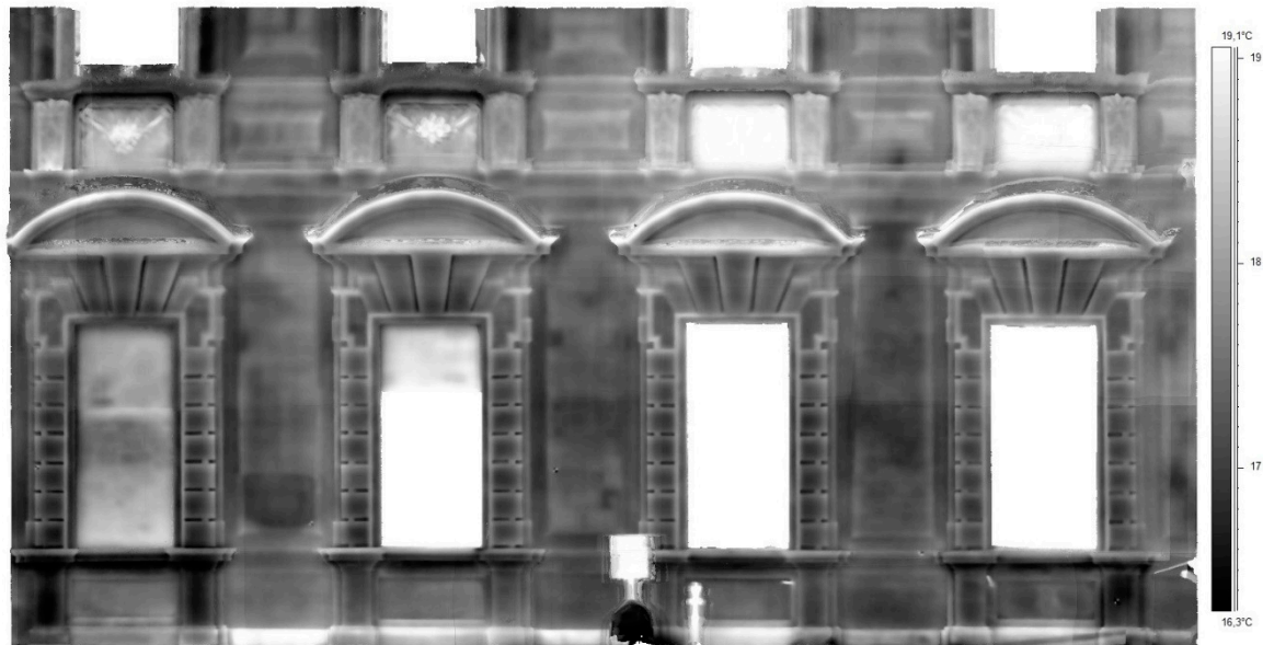
Figure 7. View of the façade's model with thermal texture.
