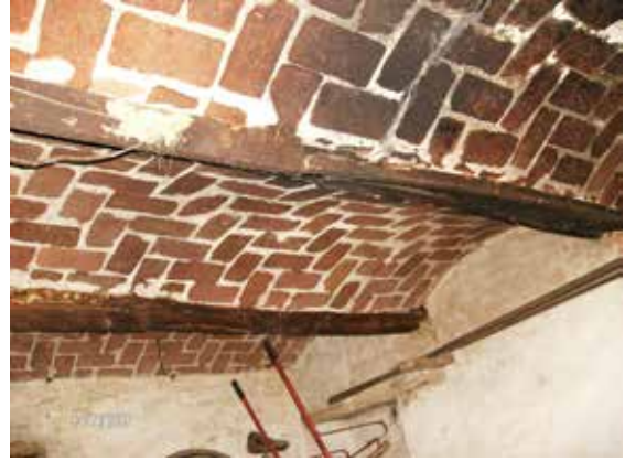
Figure 6. H-beams which support brick barrel vaults (credits Manuela Mattone)
