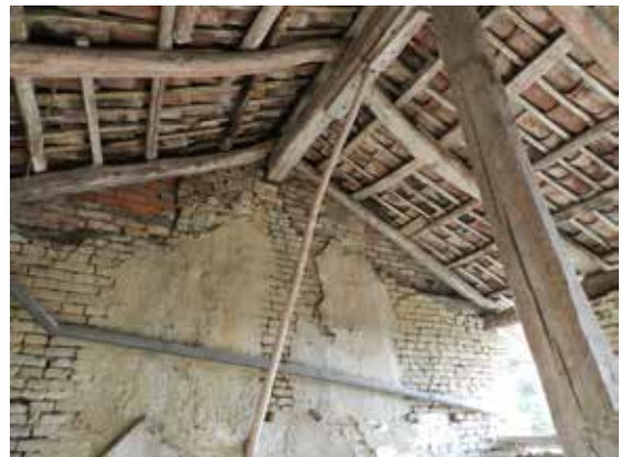
Figure 8. Wooden roof structure (credits Manuela Mattone)
