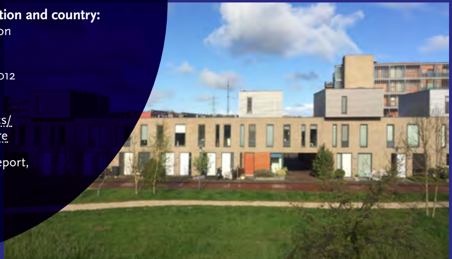
Compact suburban development – Leiden, The Netherlands
