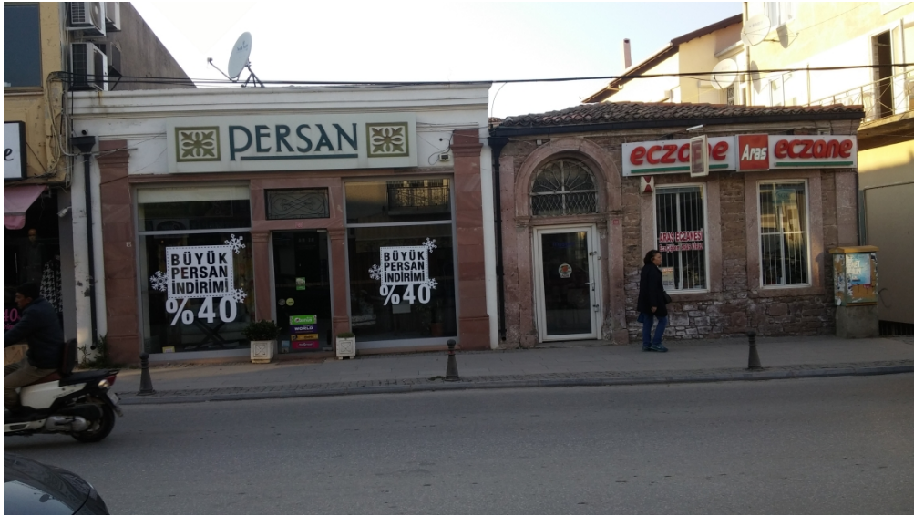
A view of converted depots
