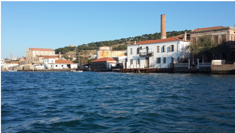
A View of the Northern Industrial Zone from the sea
