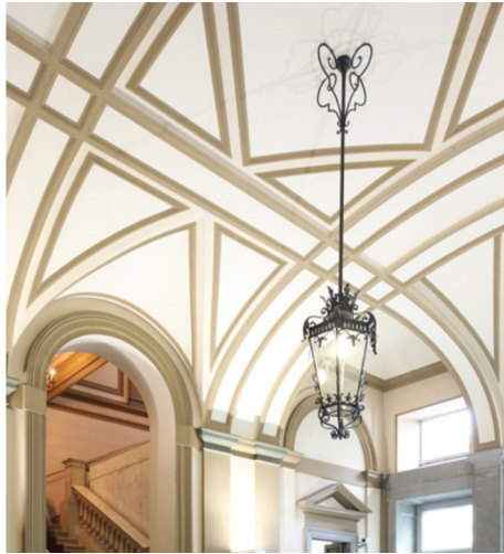
Fig. 6. Banded vault in the atrium of Palazzo Baroni di Tavigliano (photo by Marco Vitali).
