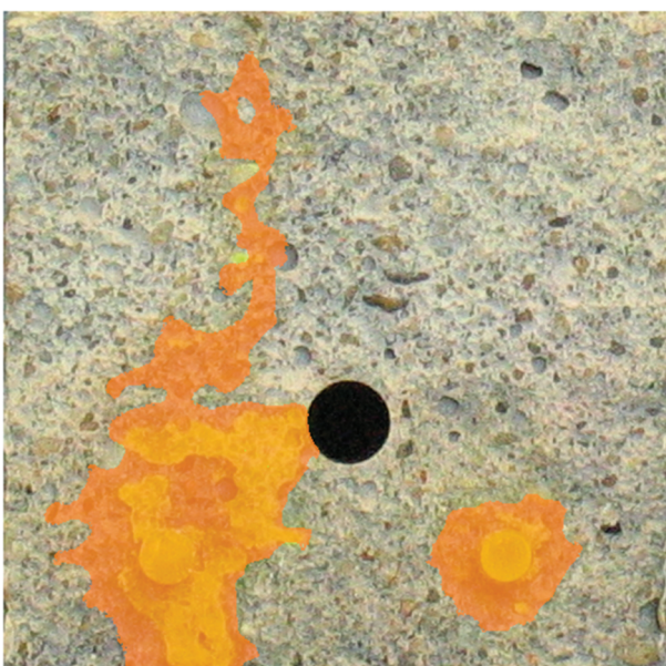
Figure 18. Crack surface ( 40 \times 40 \text{ mm}^2 ) of specimen with limited PU surface coverage. The crack mouth through which water leaked out of the specimen is oriented to the bottom, like in the water flow test.
