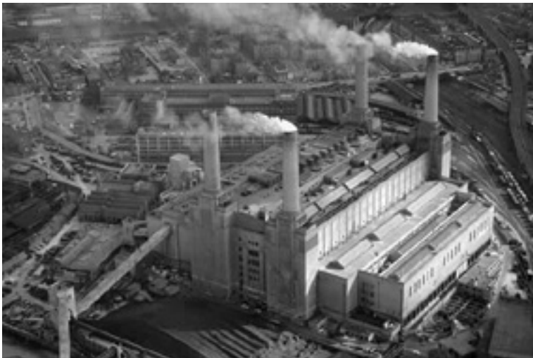
Battersea Power Station under construction and in function
