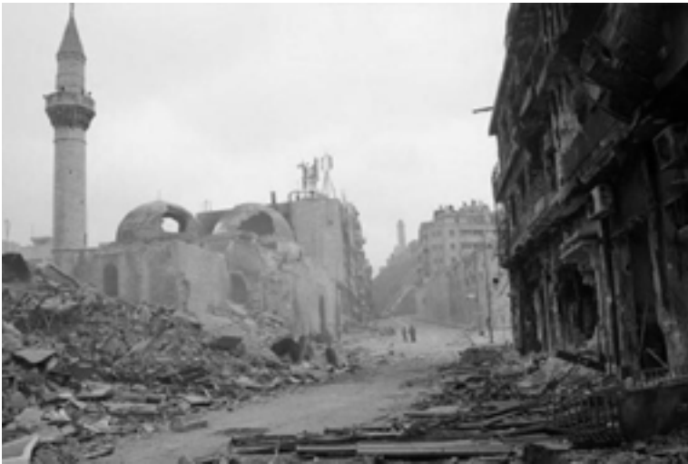
Destructions in Aleppo city, 2014
