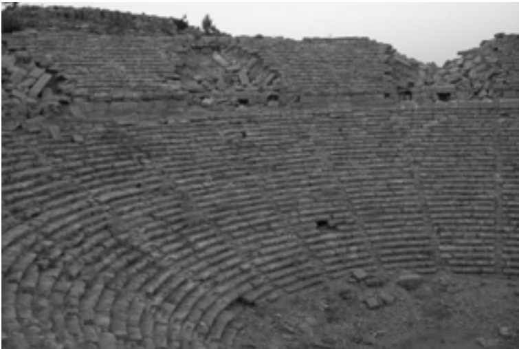
Didima and Selge: collapsed columns of the Apollo Temple and primary collapse in correspondence of the theatre cavea
