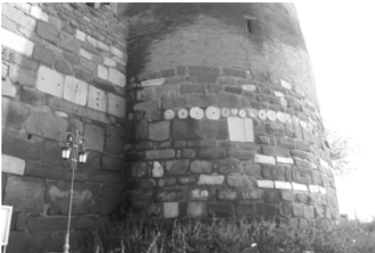
Reuse of archaeological parts in the Medieval structure
