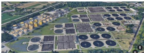
Figure 1: Photo of the WWTP.
