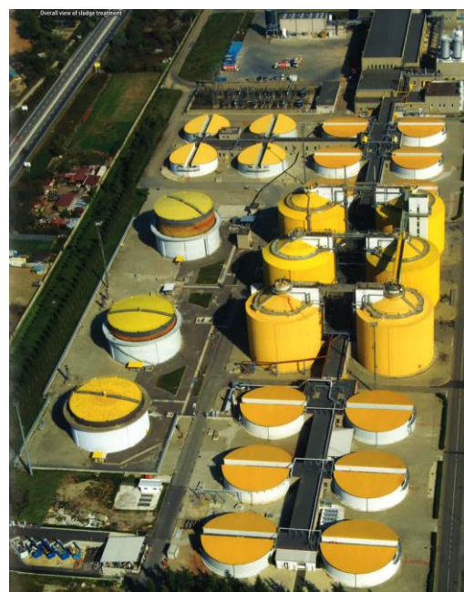
Figure 2: Photo of the sludge treatment line.
