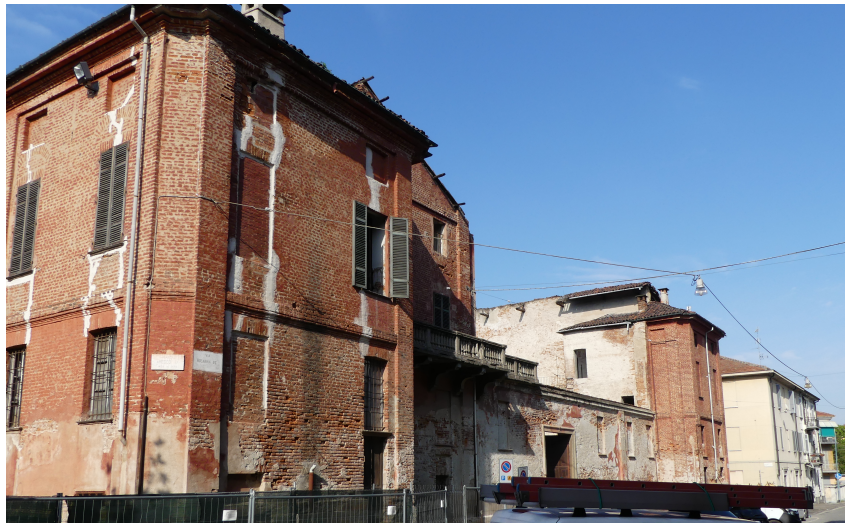
(b) Picture of the south side of the building
