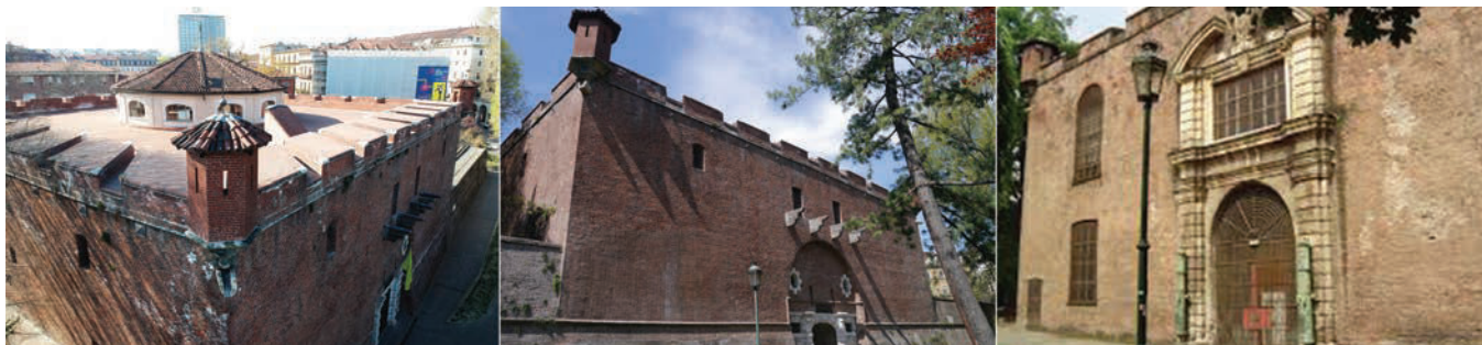
Figure 2. Aerial view (left), main entrance (centre) and rear entrance (right) of the Mastio.
