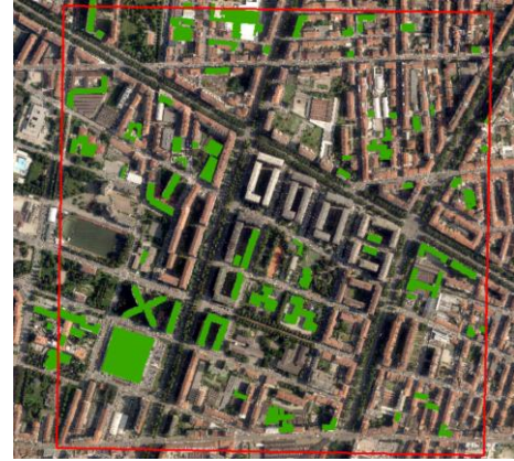
Figure 9. Potential green roofs
