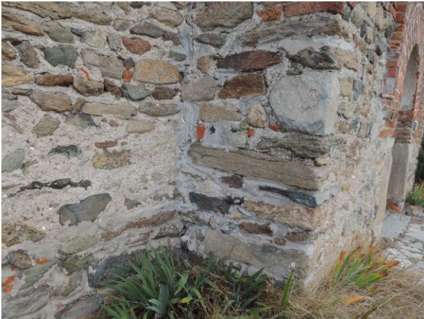
Figure 13. Building A - Grouting with cement mortar (credits Fabio Fratini).
