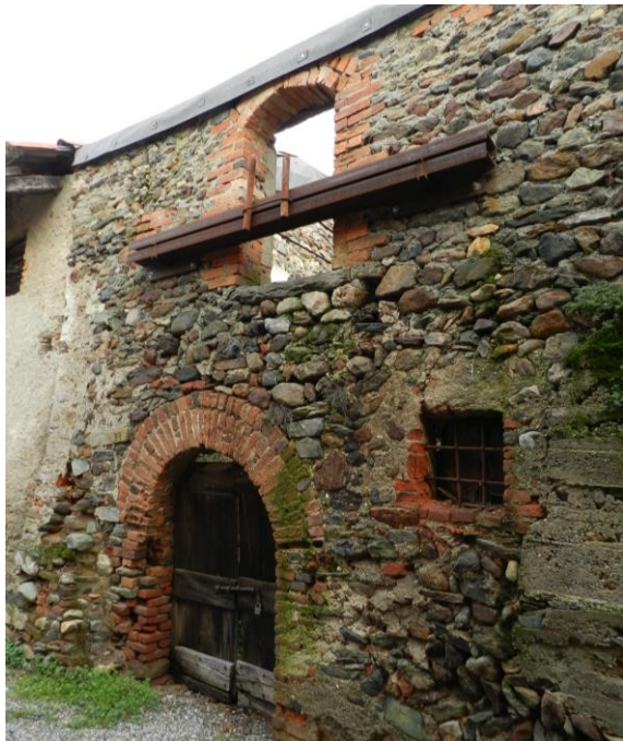
Figure 6. Building C - Temporary consolidation intervention carried out by the municipality (credits Manuela Mattone).
