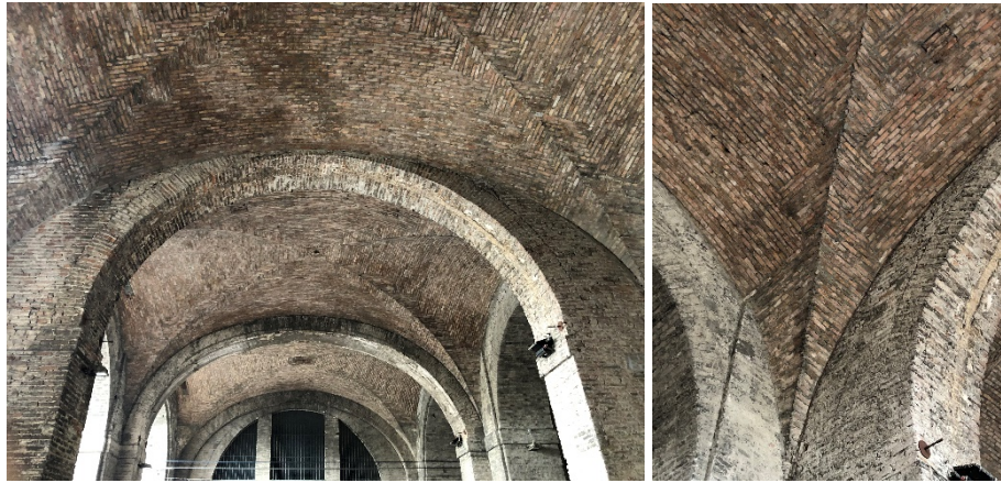
Fig 8 Pitched cross vaults in Palazzo della Pilotta, Parma, Italy: left) General view; right) detail of the corbelled bricks along the diagonal arches. Photo: Marco Alforno
