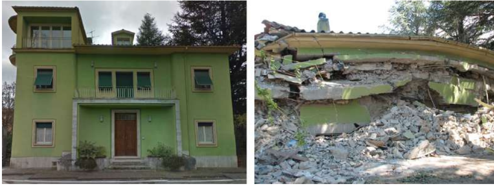
787 345 Figure 10. View of the building used as case study before and after the earthquake. 788 789 346
