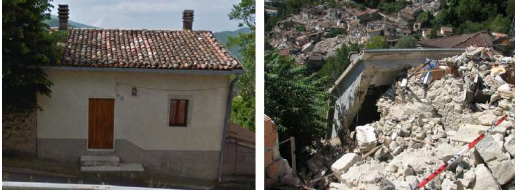
Figure 8. View of the building used as case study before and after the earthquake.
