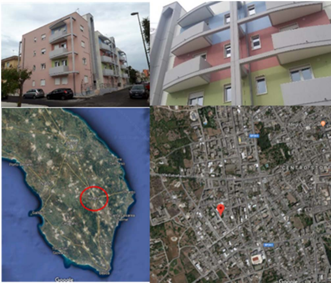
Fig. 11. New Buildings and their location.
