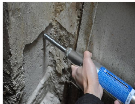
Figure 6. Constructional element identification using concrete hammer test
