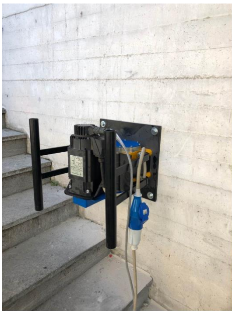
Figure 7. Application of the vibrodyne on the shear wall
