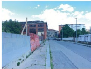
Via Carmagnola: The poor road conditions and the location of abandoned buildings make the area appear dangerous.
