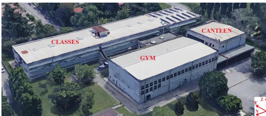
Figure 3. (a) Building overall view, (b) classes, and (c) gym building
