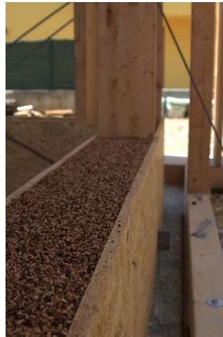
Figure 11. Cork used to drain water and for insulation purposes.
