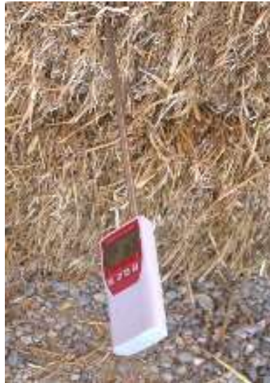
Figure 2. A straw hygrometer used to control humidity during construction. The moisture content of each straw bale is recorded.
