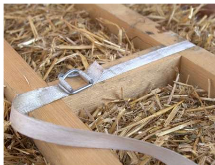
Figure 7. Fixing the bales with a composite polyester textile strap in the center.
