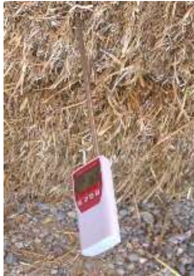
Figure 2. A straw hygrometer used to control humidity during construction. The moisture content of each straw bale is recorded.
