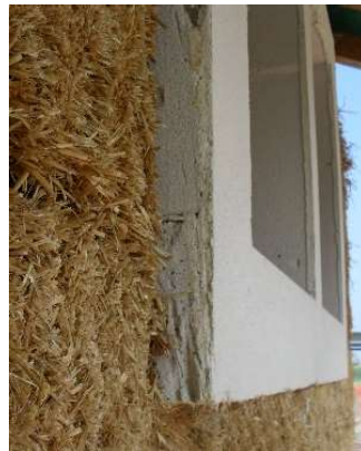
Figure 9. Edging of the windows with calcium silicate panels.
