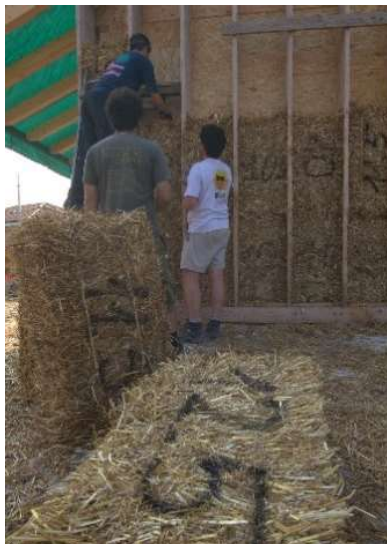
Figure 3. Dimensions and placement of straw bales: on their edges (sides), face up; flat, visible sides.
