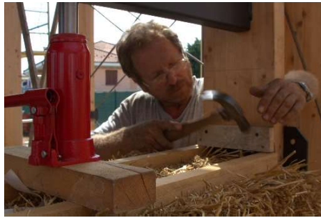
Figure 8. Compression by means of a hydraulic jack and side fixing with screws.
