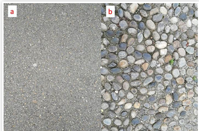
FIGURE 4 Asphalted (a) and cobblestoned (b) road surfaces.
