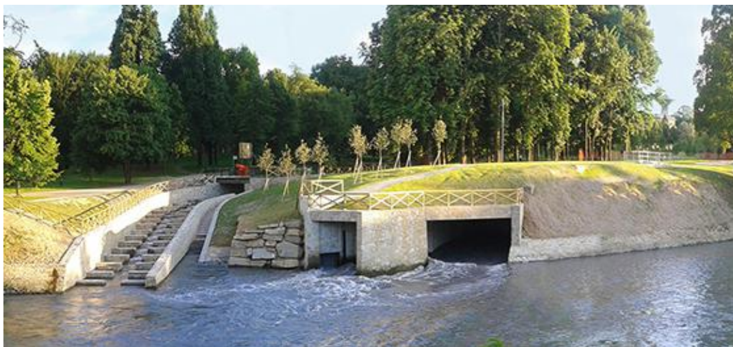
Fig. 5. Mini-hydro power plant installed in the urban park of Pellerina (Authors, 2018).
