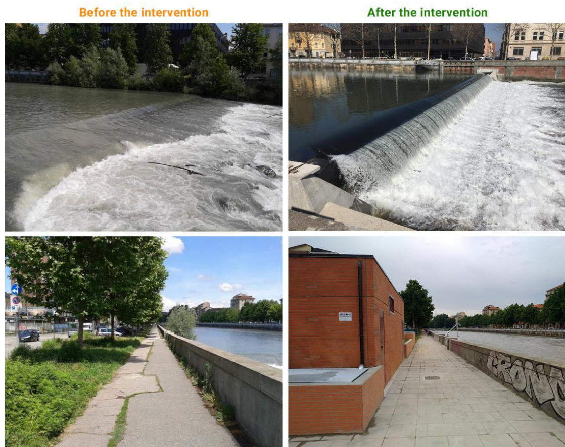
Fig. 11. The status of the Regio Parco check dam and the pedestrian sidewalk before and after the installation of mini-hydro power plant. The intervention includes also the requalification of the right riverbanks (Authors, 2018).
