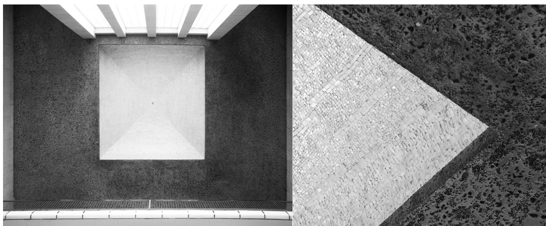
Figure 10. Steining on the ceiling of the main entrance of the University of Iceland. The central vault is rendered with calcite fragments, the surrounding portion with obsidian on a blue-cement field. Photos by Sofia Nannini.
